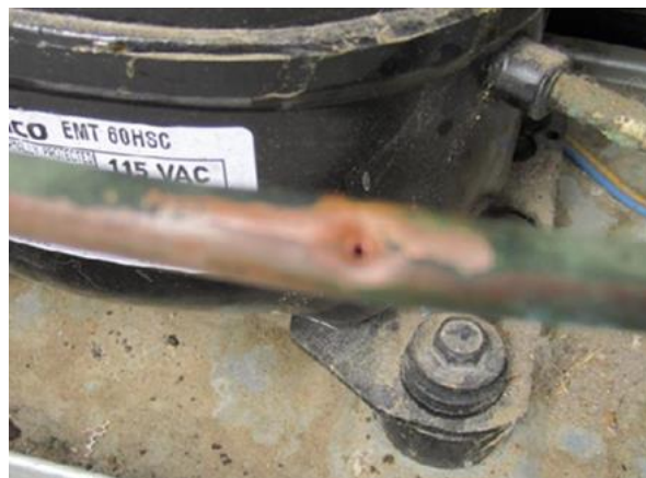
Figure 1: Drained Refrigerant lines will have a puncture mark.
