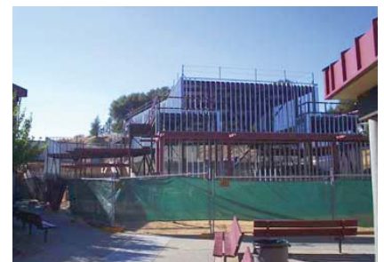
Construction of Performing Arts Center
