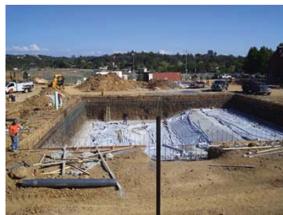
Aquatic Center Pool Construction
