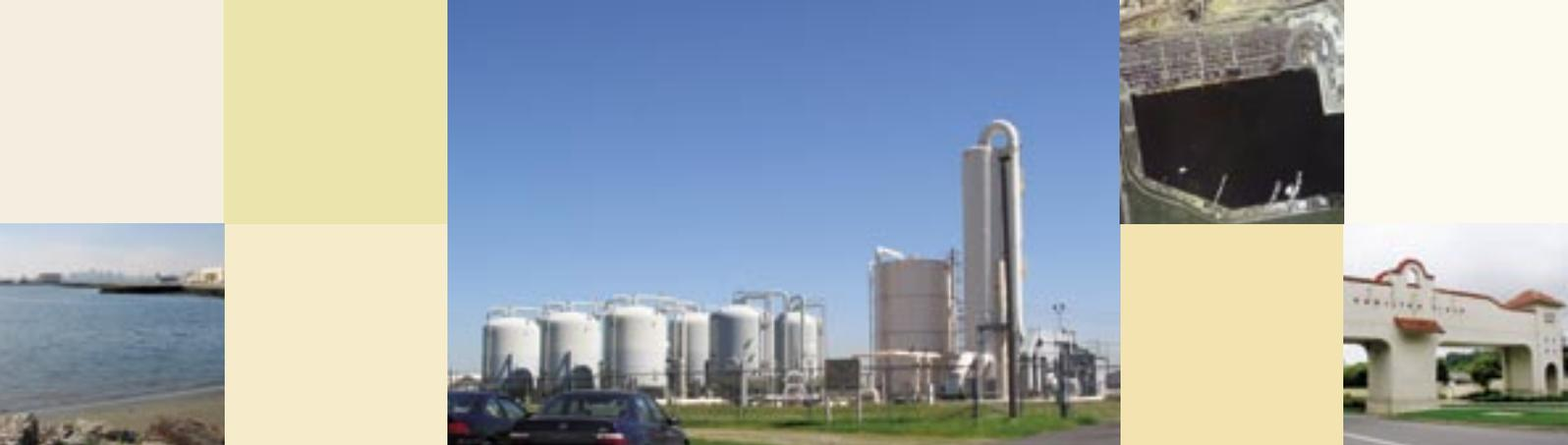
Dual Phase Treatment System, that combines Soil Vapor Extraction systems with groundwater treatment systems, used to treat groundwater contamination at McClellan Air Force Base.
