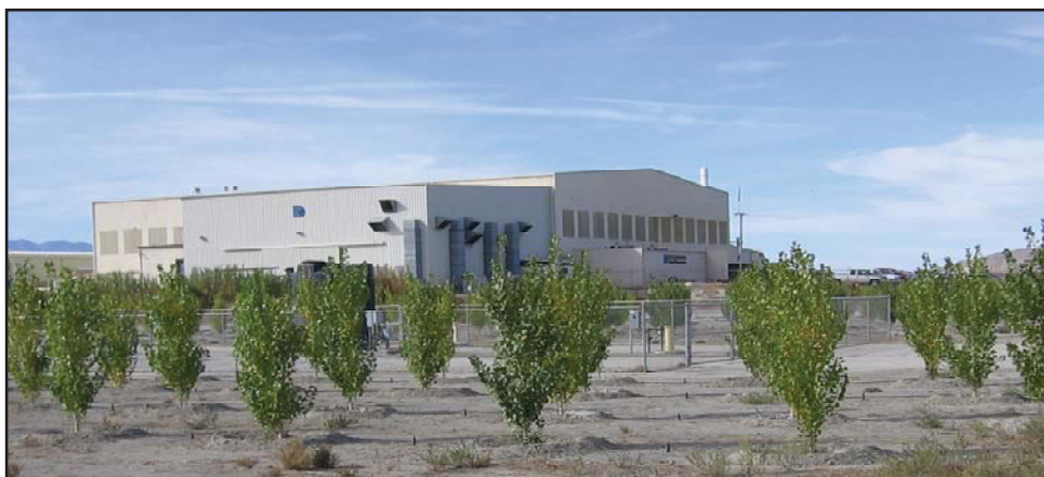
Photo of the facility viewed toward the southwest
