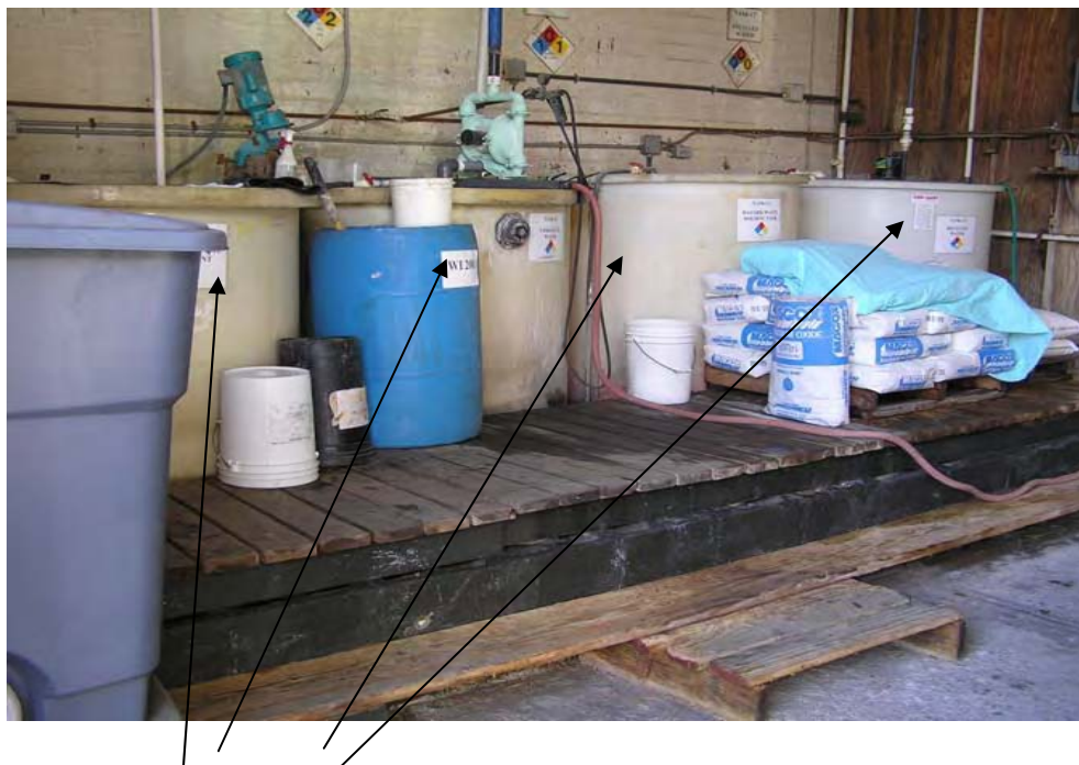
Tanks and containers used to hold and treat hazardous wastes
