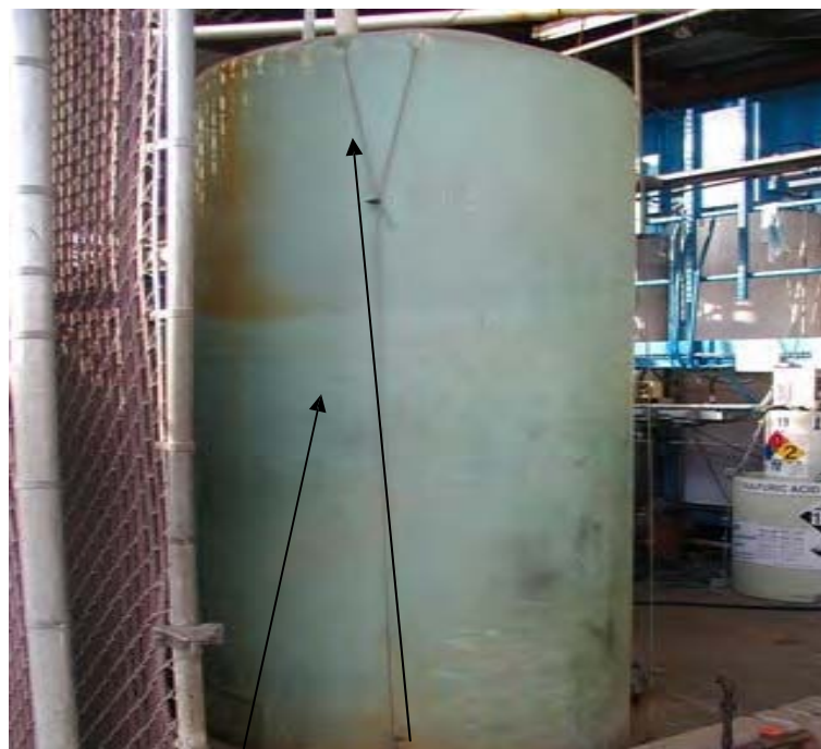
Back-wash holding tank with proper seismic anchoring
