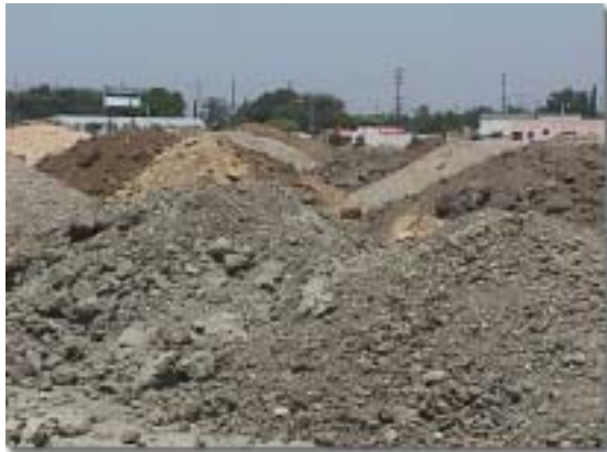
Excavated soil at the Southeast Middle School and High School site in Los Angeles.
