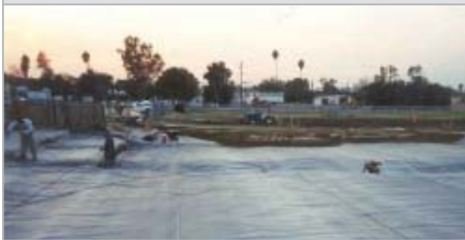
A high-density polyethylene (HDPE) liner prevents residual contamination from rising to the surface.
