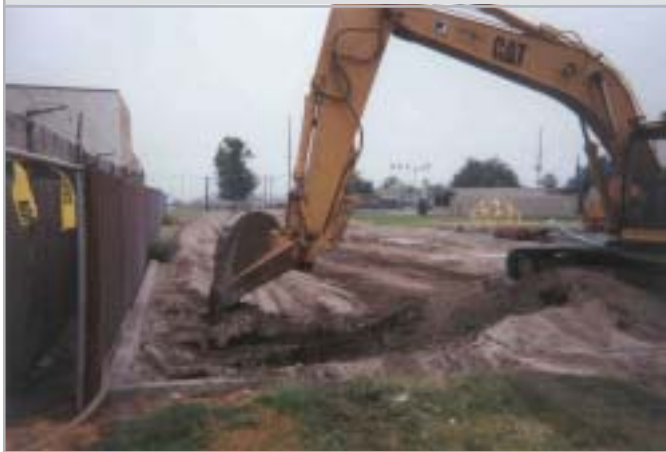
Excavating sand from the playground area as requested by the San Bernardino City Unified School District.
