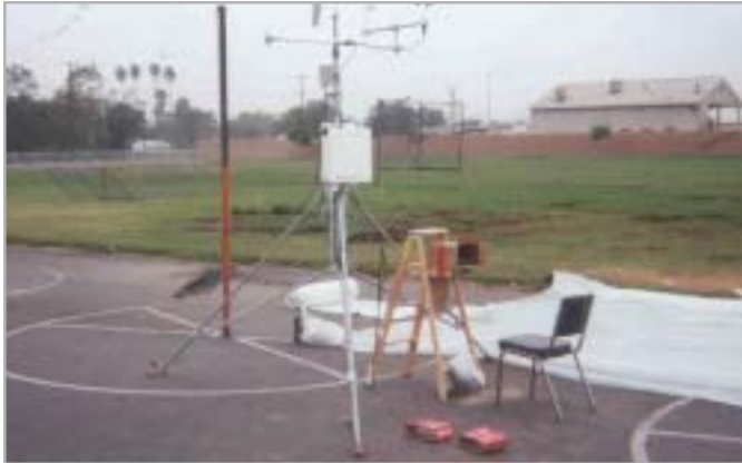
A meteorologic station was erected on the Burbank Elementary School property during the removal to monitor weather conditions including wind speed and direction.
