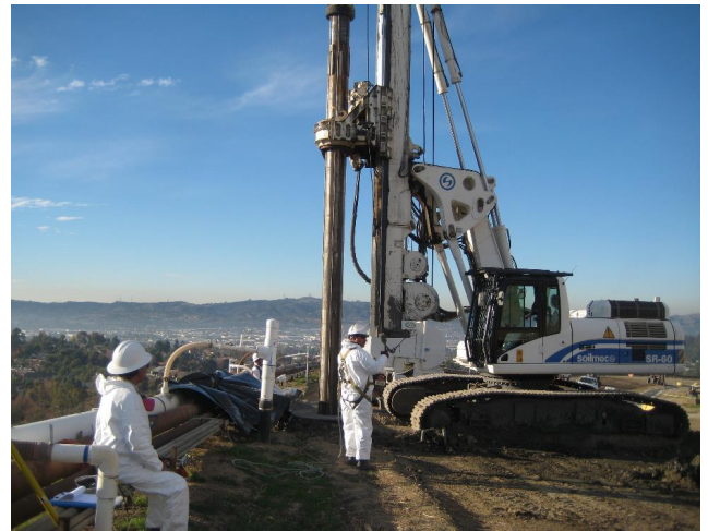
Installation of Landfill Gas Wells
