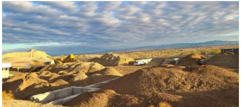
Photograph 3: Soil Processing Yard - more than 12,600 cubic yards of excess soil was generated during Phase 1 construction, of which 90% was reused onsite
