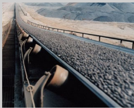
Belt conveyor (on grade)
