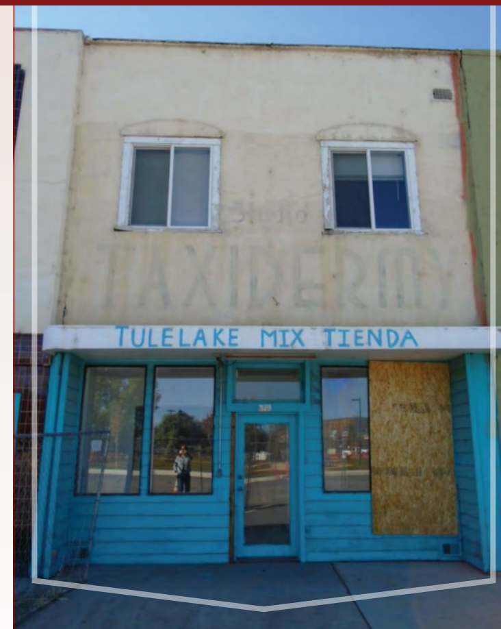
Mix Tienda Building, City of Tulare
