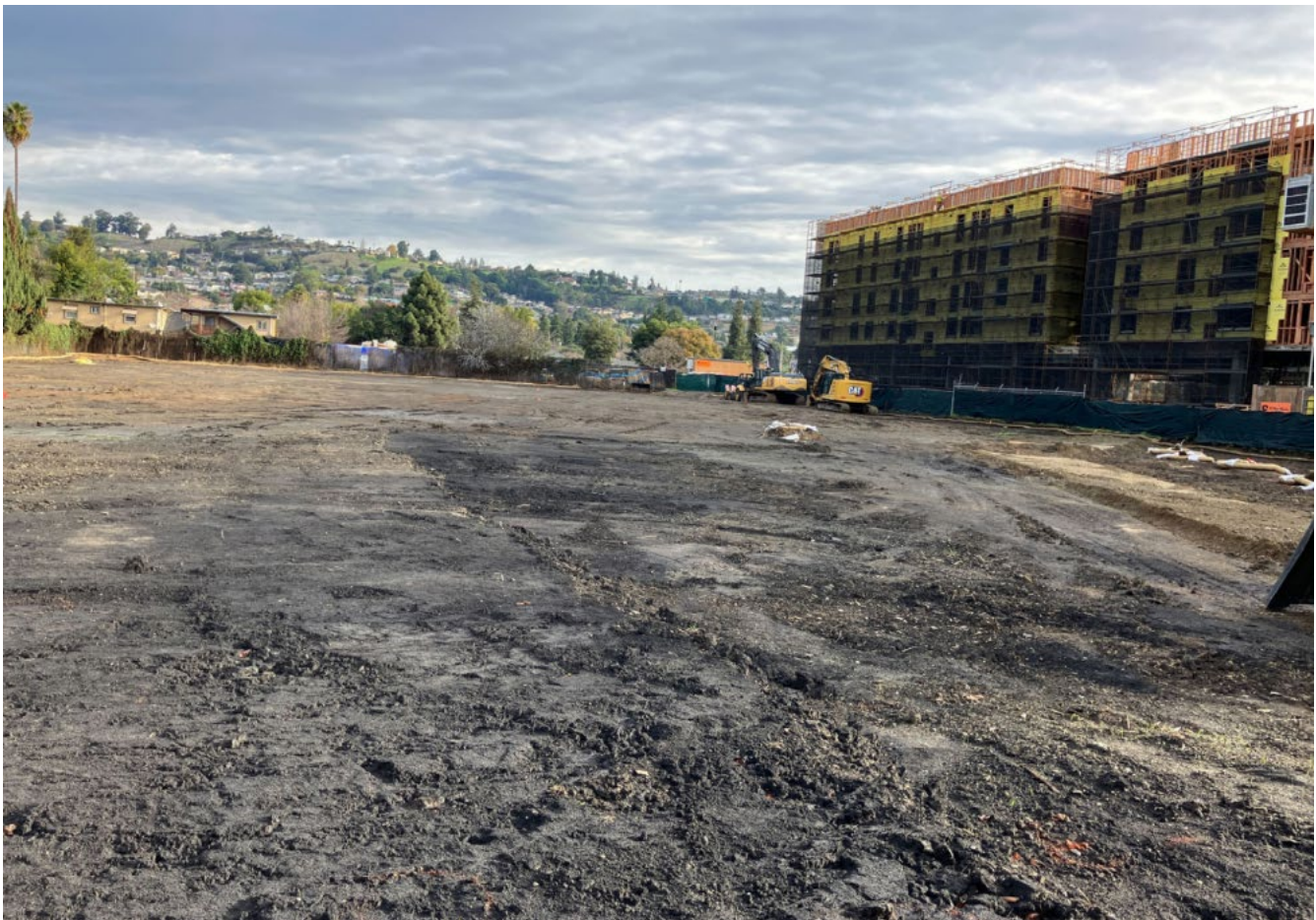
East 14th St. Park site after excavation of contaminated soil.
